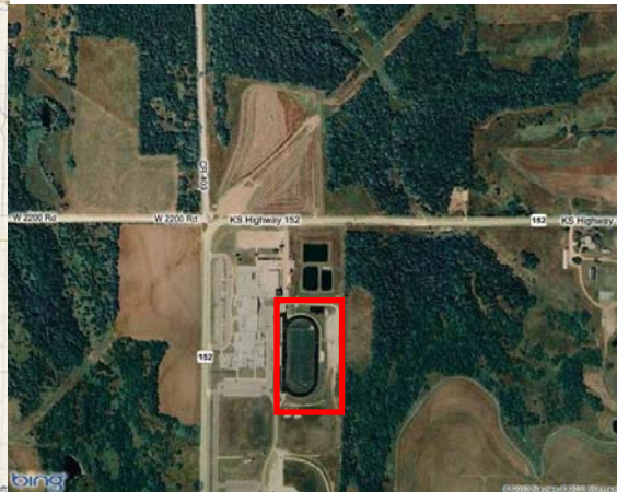
Figure 2. Aerial of Project Location
